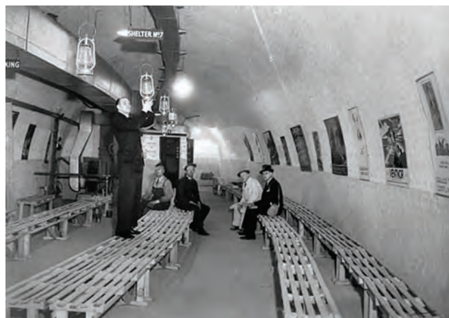
The upper level of the King William Street shelter in 1940. This has now been demolished
